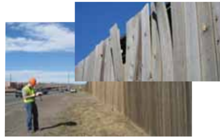
Project builds new/repairs aging noise walls.
