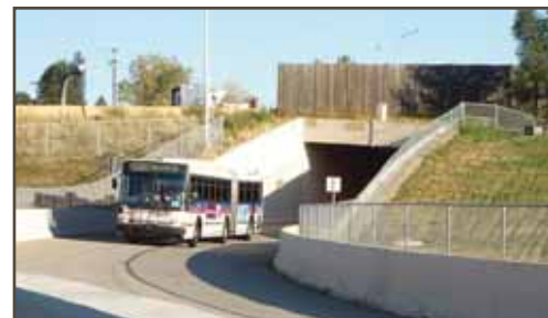
To the north, project links to Wagon Road Park N Ride via direct-connect tunnel.
