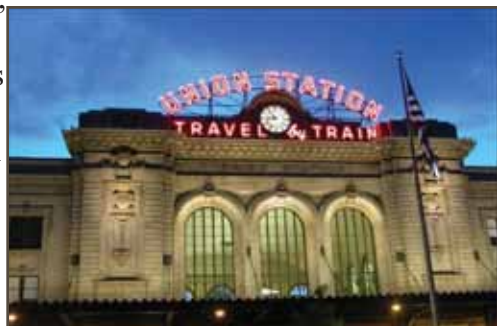
To the south, project connects to Denver Union Station in downtown Denver.
